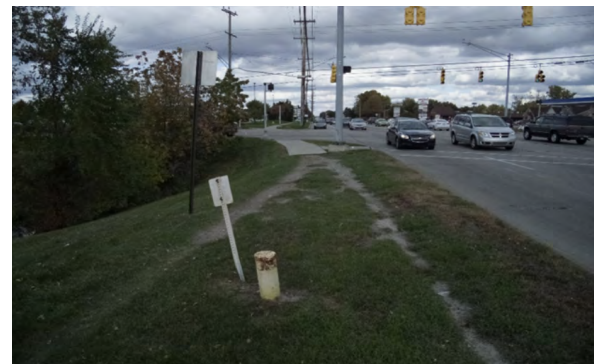
Designing for the needs of a particular area can lead to more effective and cost-efficient infrastructure.
