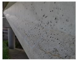
Longitudinal and alligator cracking may be caused by alkali-aggregate reactivity and generally occurs on beams exposed to direct sunlight.
