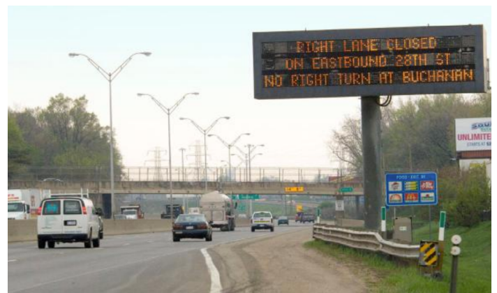
Dynamic message signs are one element of MDOT's ITS statewide network. They rapidly convey important information about unexpected or changing conditions.
