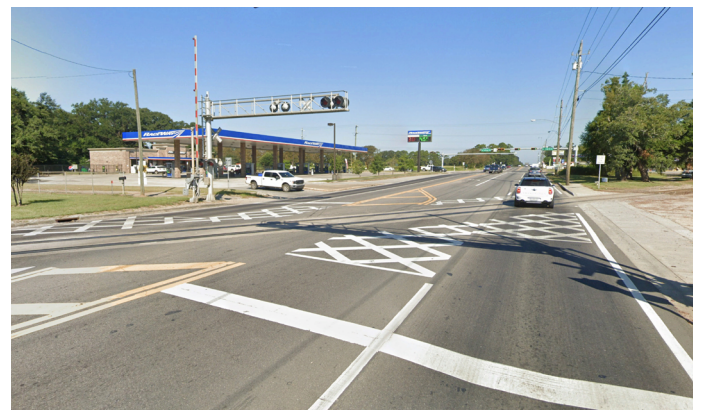
Train crossings with short storage can be challenging for drivers. Additional road markings and signage can reduce crashes.
