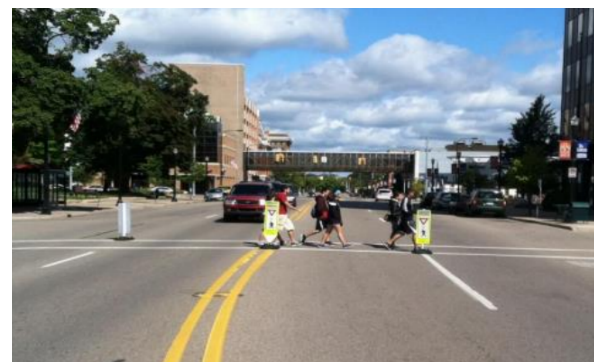
MDOT strives to integrate the needs of pedestrians and bicyclists into all facets of transportation design.
