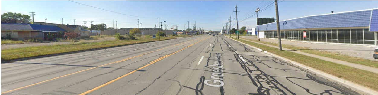
Figure 23. M-97 Google Street View
