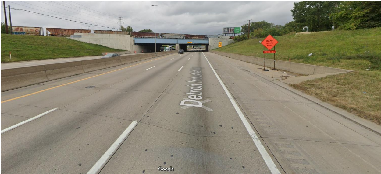
Figure 32. I-94 Google Street View
