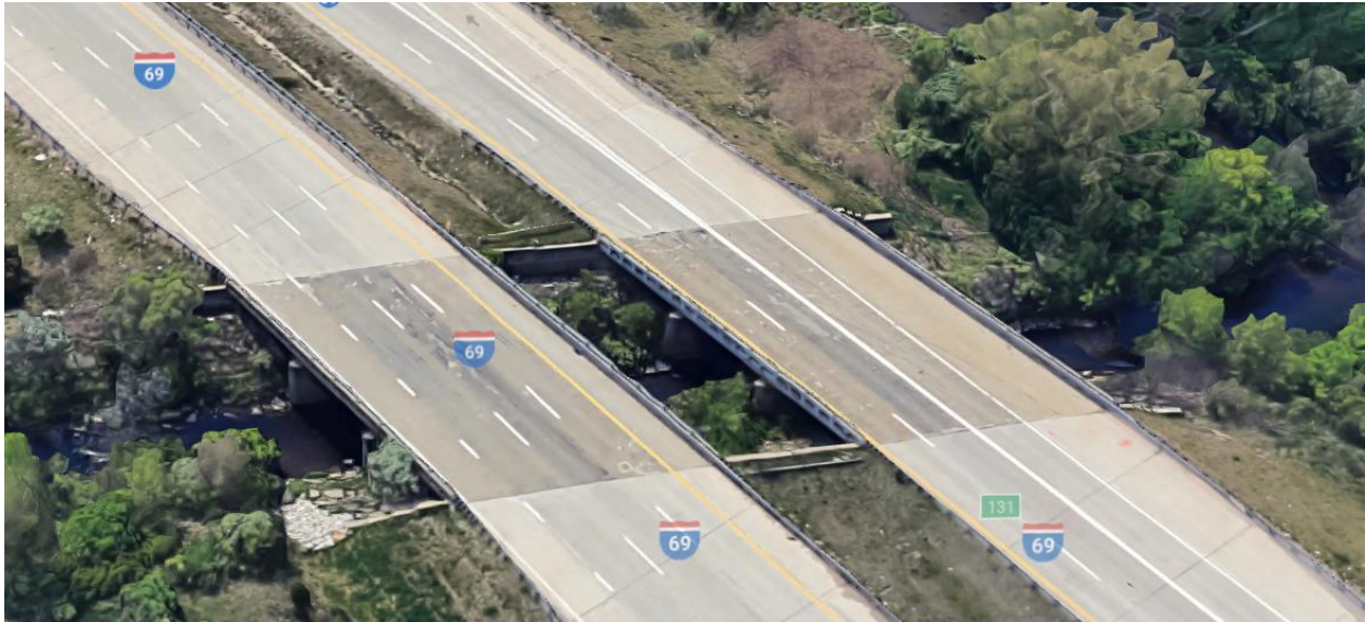
Figure 34. Google Earth 3-D Screen Capture of Bridges ID 25125042000B023 and 25125042000B024 Along I-69 lxxii
