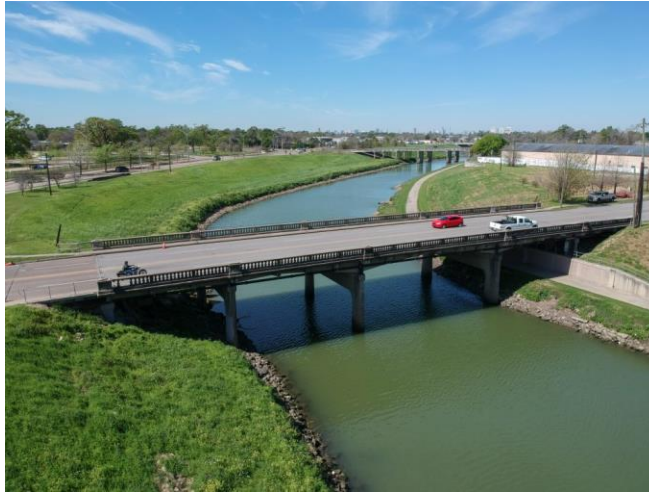
Figure 37. Bridge Deck in Houston, Texas lxv
