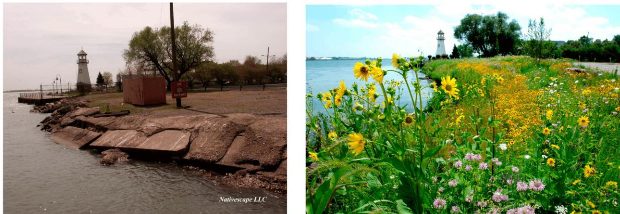
Figure 30. Living Shoreline at Rogue Power Plant, Michigan (Left–Before, Right–After) lxx
