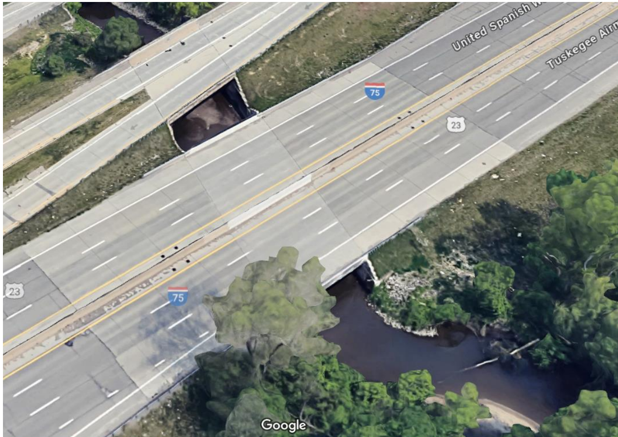
Figure 36. Google Earth Screen Capture of Bridge ID25125031000B030 on I-75 lxxiv
