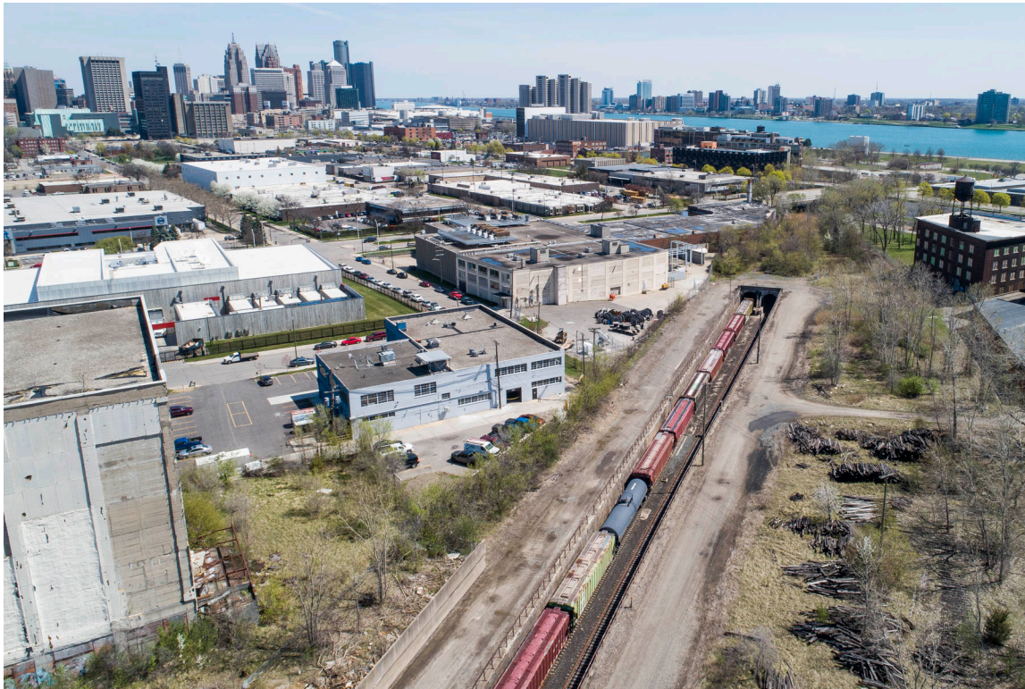
Figure 51. Canadian Pacific Detroit-Windsor Tunnel
