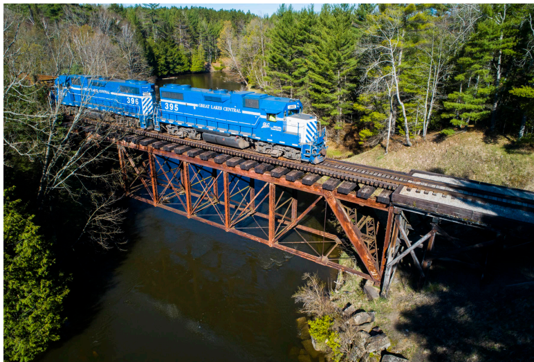
Figure 48. MDOT-Owned Manistee River Bridge
