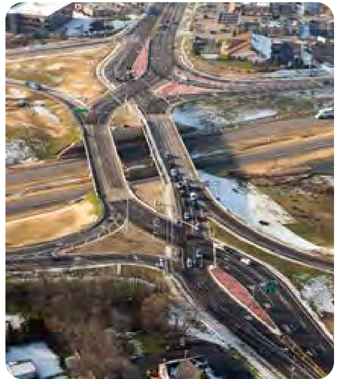
Diverging diamond interchange, Kent County
