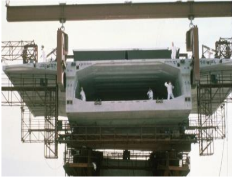
104 Prestressed Closed Web/Box Girder (Segmental)
