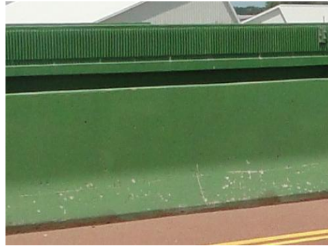
521 Concrete Protective Coating
