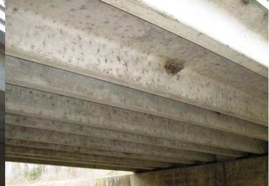
109 Prestressed Concrete Open Girder (Precast Double T)
