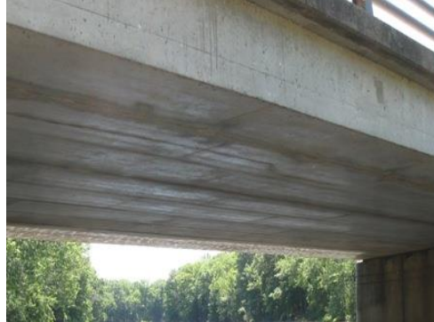
823 Prestressed Concrete Box Beams (Side-by-Side)
