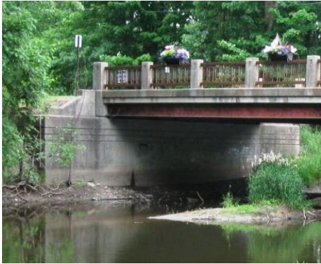
215 Reinforced Concrete Abutment
