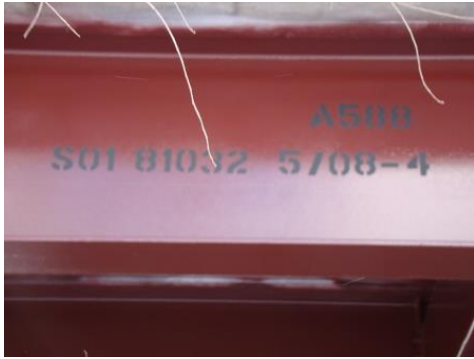
515 Steel Protective Coating
