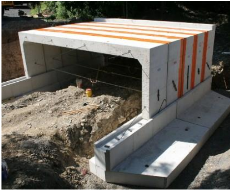
3-Sided Concrete Box Culvert
