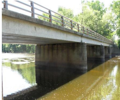
210 Reinforced Concrete Pier Wall
