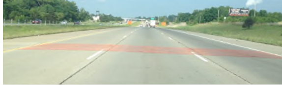
Exhibit 6-16 Temporary Rumble Strips in Advance of a Work Zone
