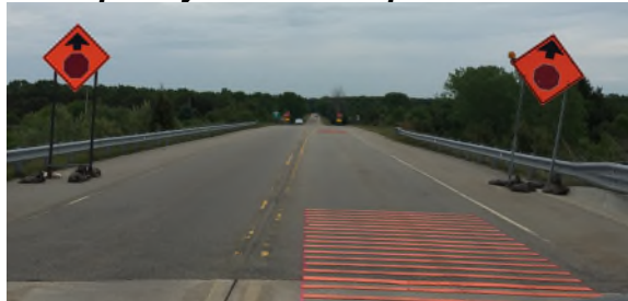
Exhibit 6-17: Temporary Rumble Strips in Advance of a stop sign
