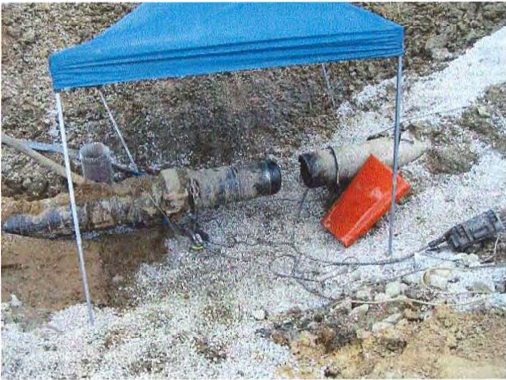
Image 2(004) : Air-gapped line, and trench.
