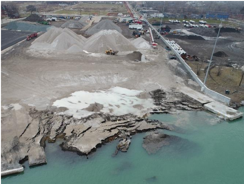
Photograph 2 – Taken by EGLE (December 6, 2019)
