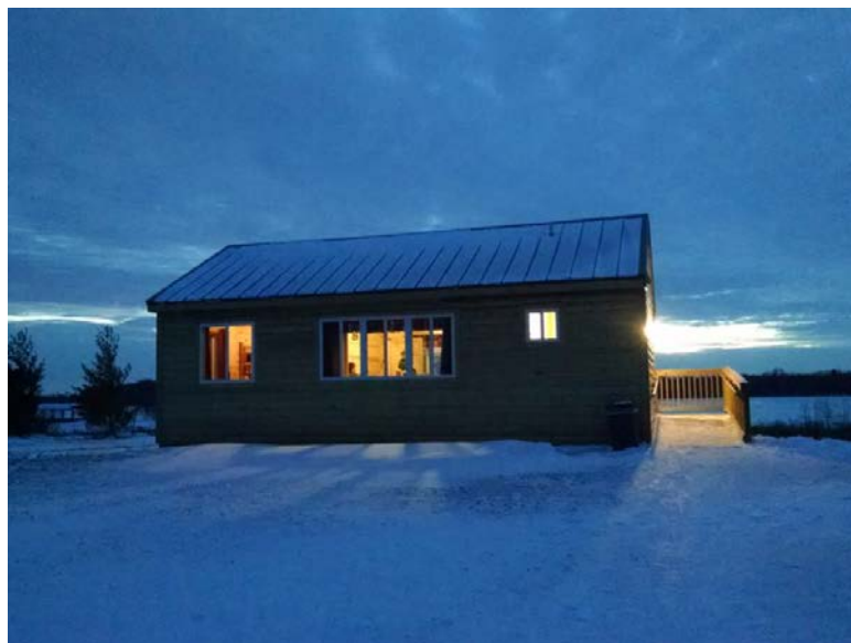
A modern cabin was constructed in the park in 2014
