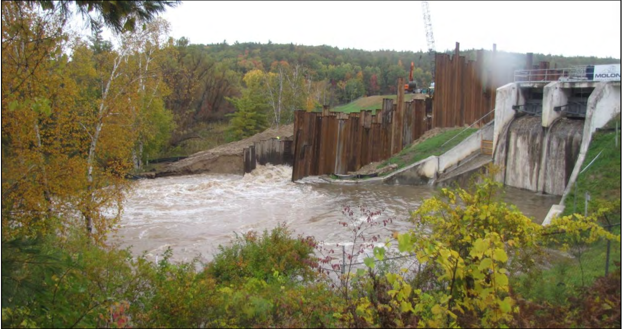
Figure II-6. Photo of TDS channel with turbulent flow from boil Photo courtesy of AMEC
