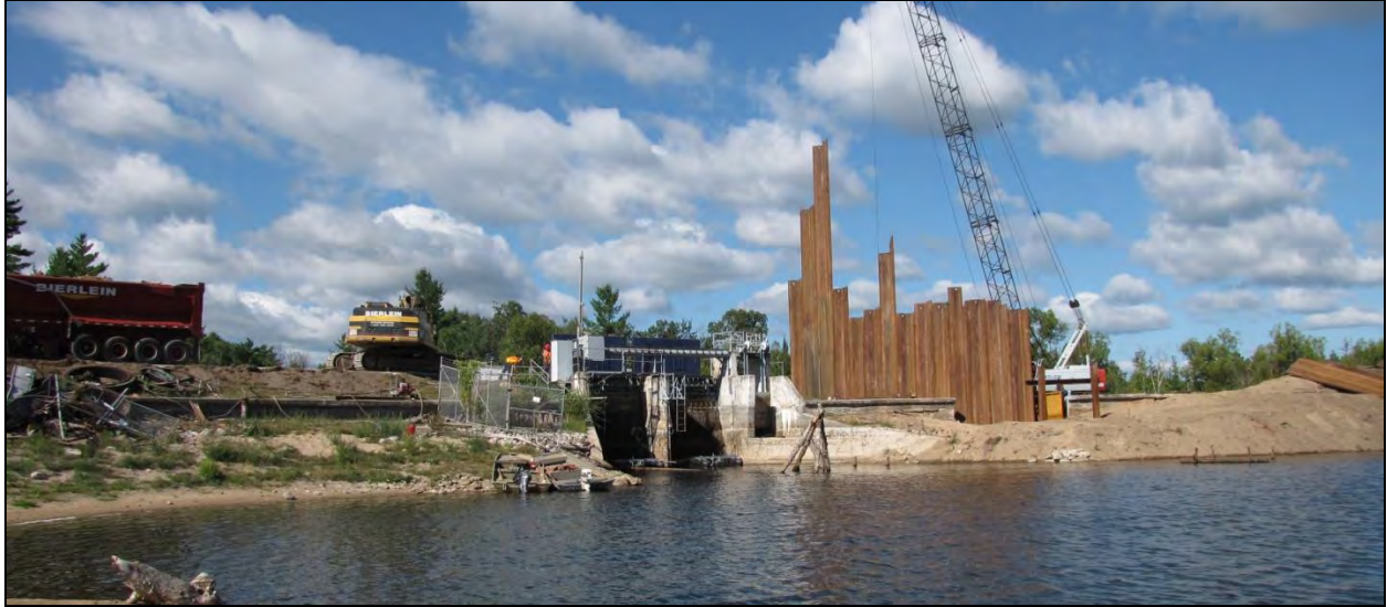
Figure II-2. Photo of the dam during TDS construction Photo courtesy of AMEC
