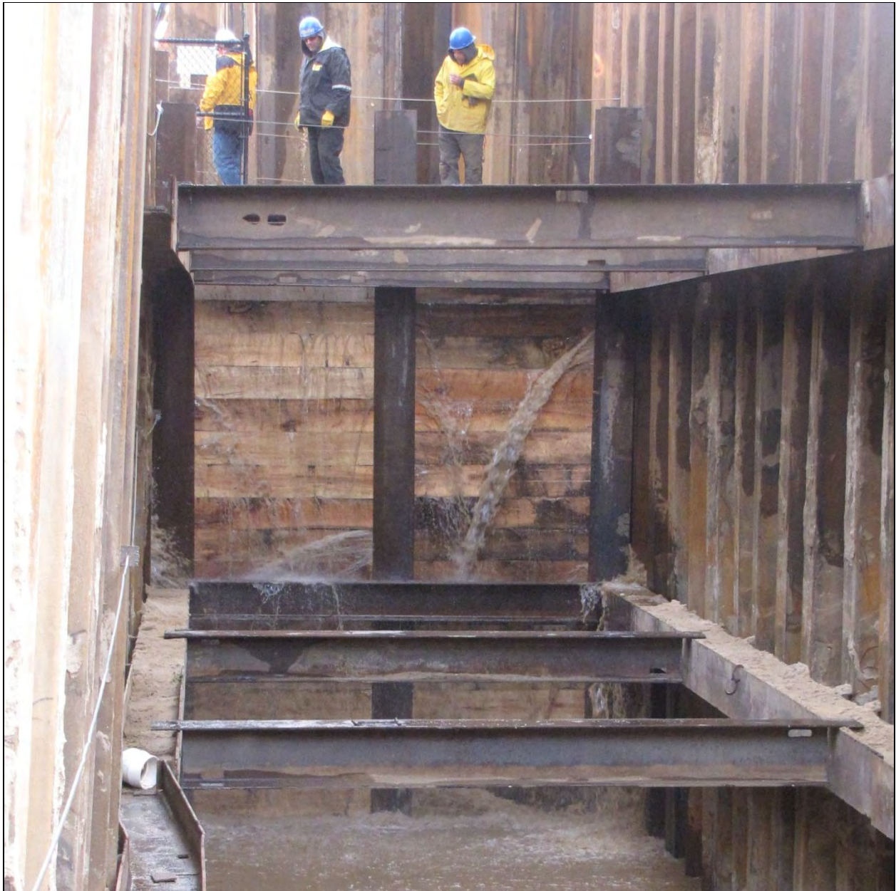
Figure II-4. Photo of TDS stoplog weir at first testing Photo courtesy of AMEC
