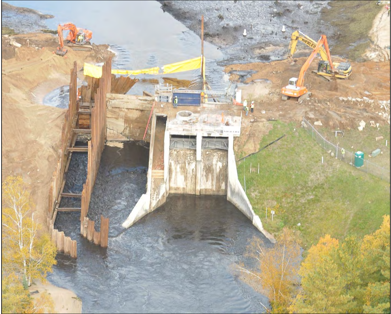
Figure II-7. Photo of the dam and TDS after complete failure Photo courtesy of John Russell, Great Lakes Imaging
