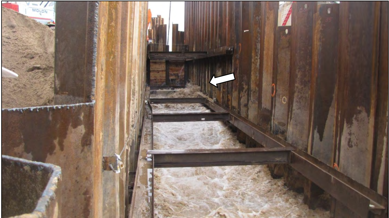
Figure II-5. Photo of TDS channel at initial boil formation (arrow indicates boil location) Courtesy of AMEC
