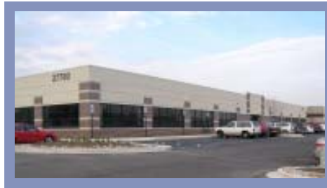
MDEQ's District Office in Warren is LEED certified.
